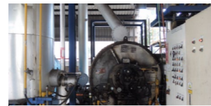
Before the replacement
