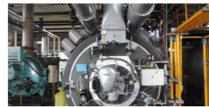
After the replacement
